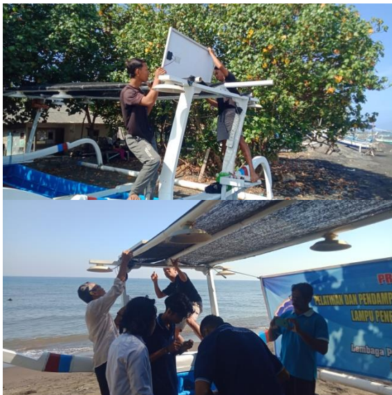
Gambar 6. Pemasangan panel surya 100 WP
